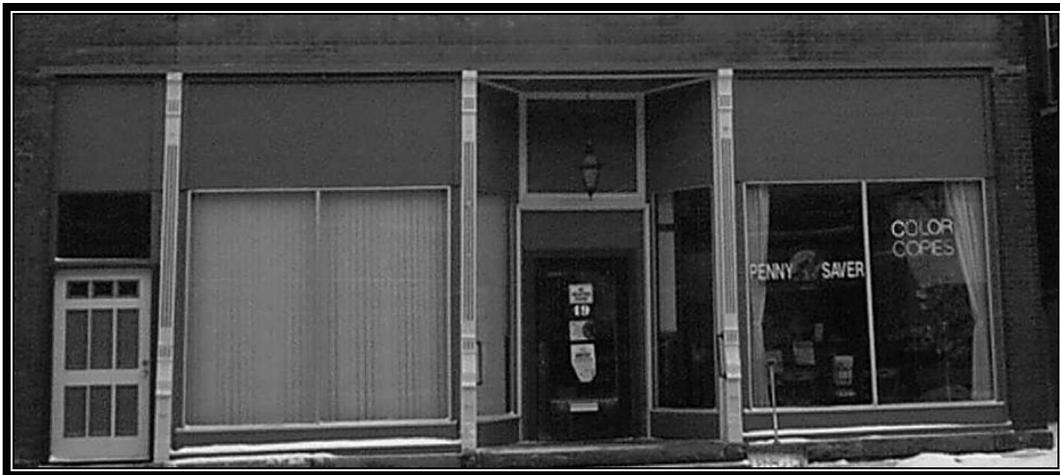
**#Don't reduce the size of storefronts or other windows by filling original openings with non-transparent construction.**
