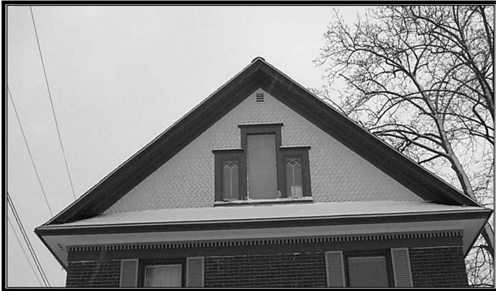
**#Pediment – Gable treatment where a triangle is formed by the two raking cornices and a continuous horizontal cornice at the base of the gable.**
