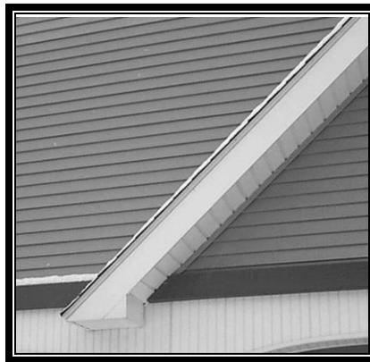
**#Modern boxed soffit – Inappropriate for pre-1950 buildings. Soffit is often level to roof slope.**
