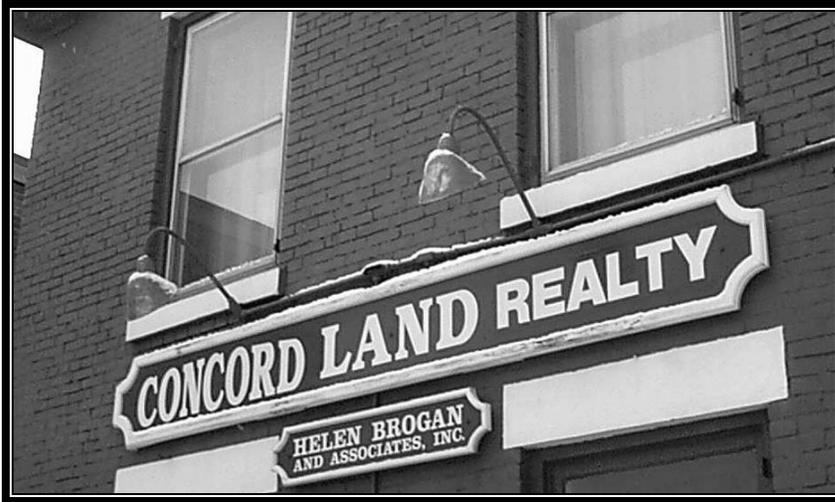
**#Gooseneck fixtures are designed to direct light toward the sign and produce little glare**
